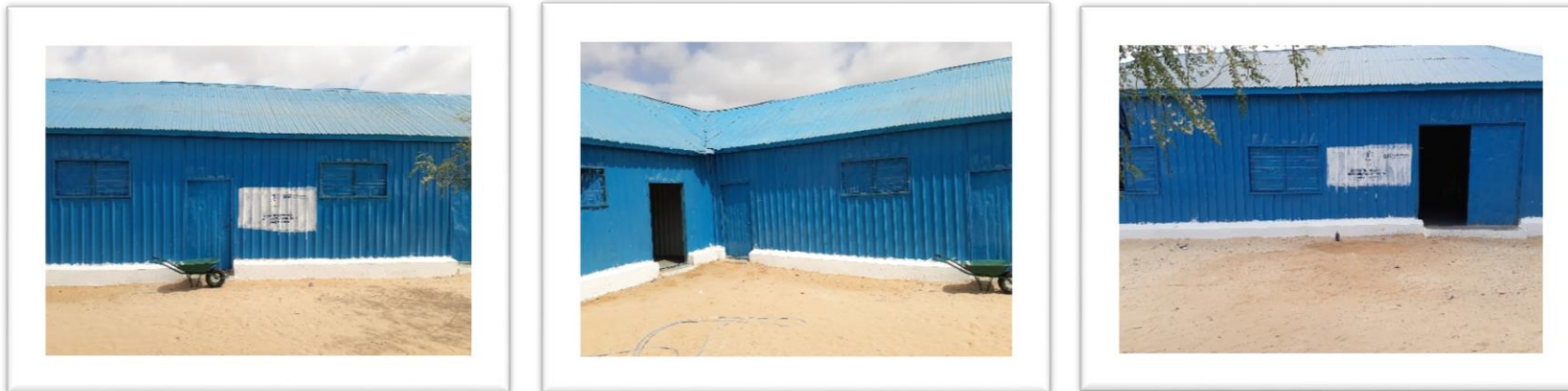
PHOTOS – BUILDING OG CLASS ROOMS, COMMUNITY CENTER AND OFFICE
